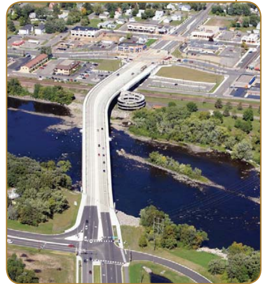
4.8 million pounds of steel were used, with the longest span at 295 feet in length.
