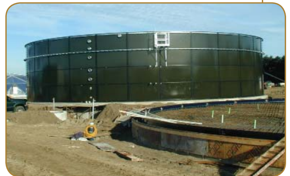
Sludge Storage Tanks
