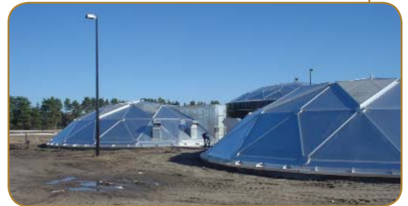
Dome Covers over Final Clarifiers
