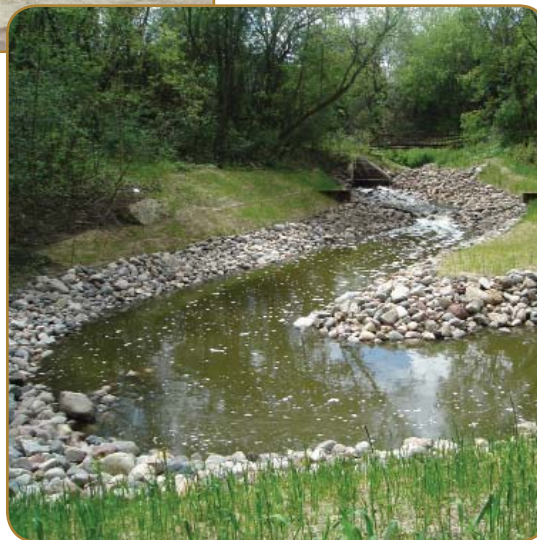
Rock riprap was installed along the banks to prevent erosion.
